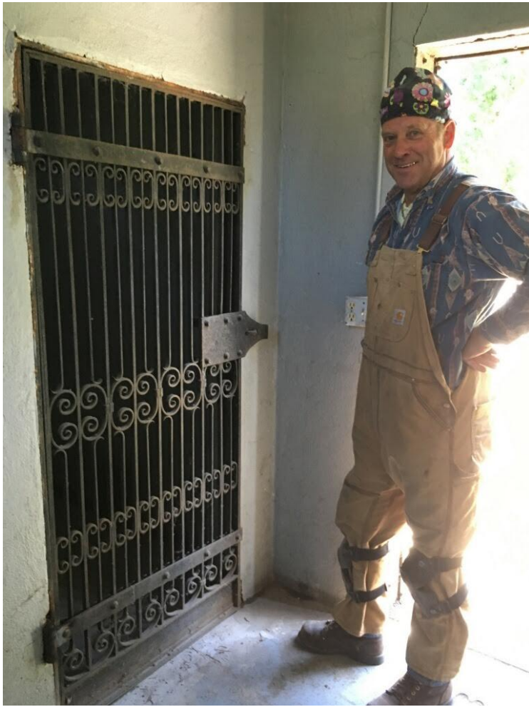
Reed Price and a repaired jail door.
