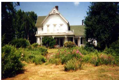
Condition of the Zimmerman grounds and house when the society took possession in 1995
